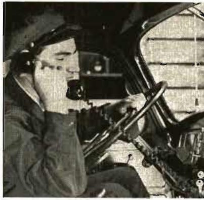
W.E. f-m telephone service system, installed by Bell System.
